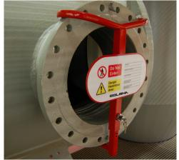
Our confined space entry barriers are designed to physically prevent unauthorised access to manway holes and vertical ladders.
